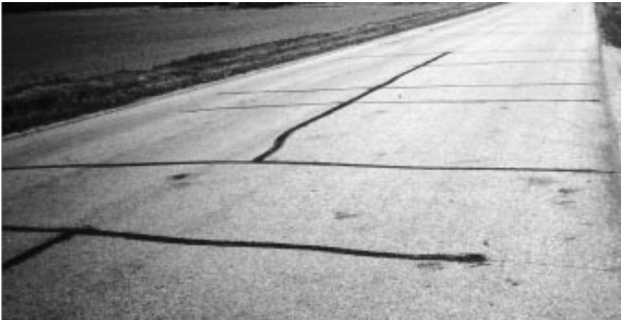
▼ Open crack, 1/2" wide; adjoining pavement sound.
