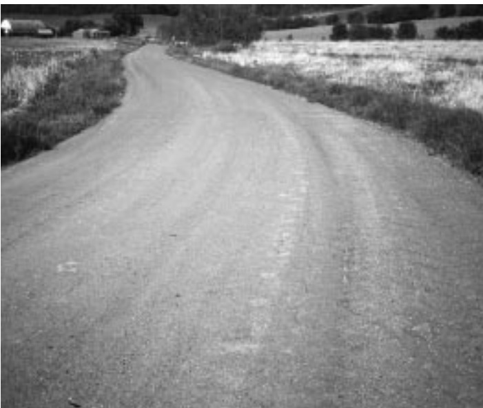
▲ New cold mix surface.
