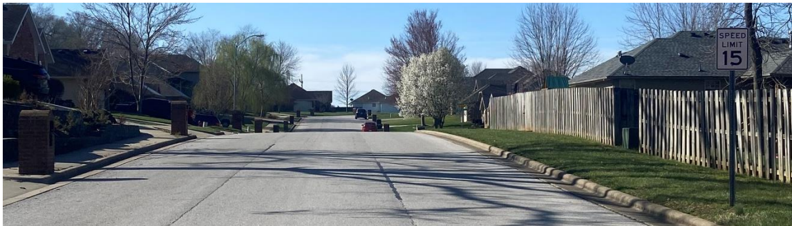
Figure 6: Site Photo - SB South of Welch Drive
