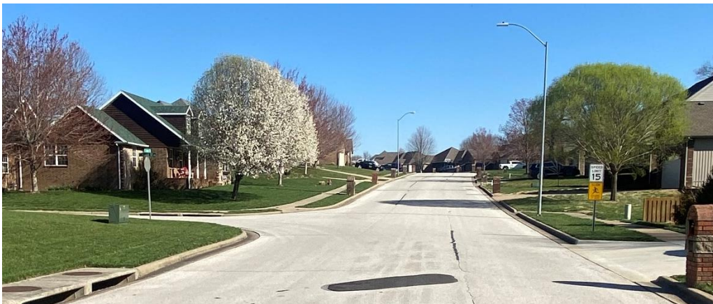
Figure 7: Site Photo - NB at Welch Drive
