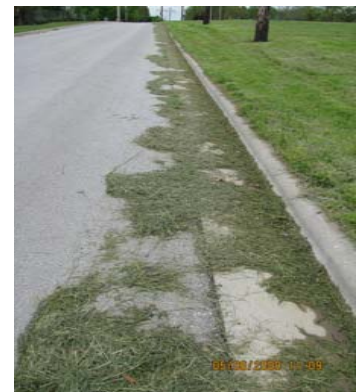
Grass in the street gutter headed for the storm sewer and eventually to the river.
